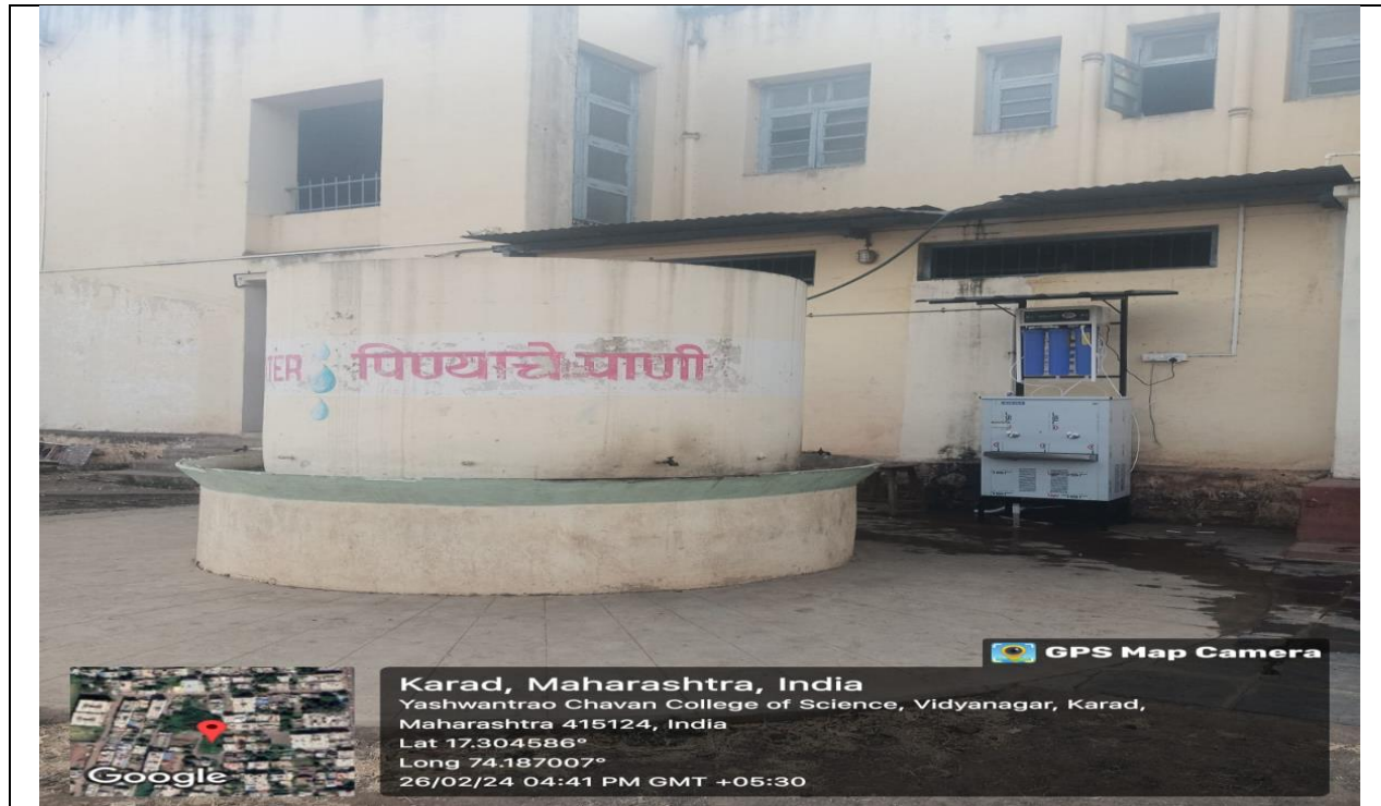
RO+ UV Water Purifier facility at Main Building
